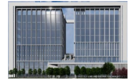
C1/C2 Building, Shui-Nan Campus
