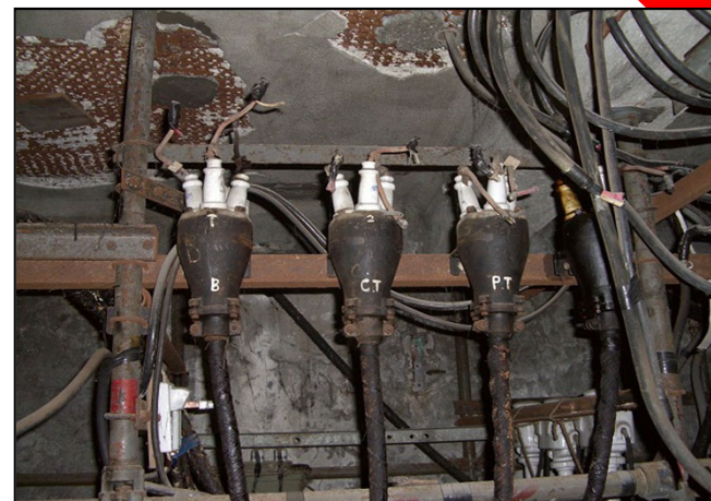
Aging substation equipment
