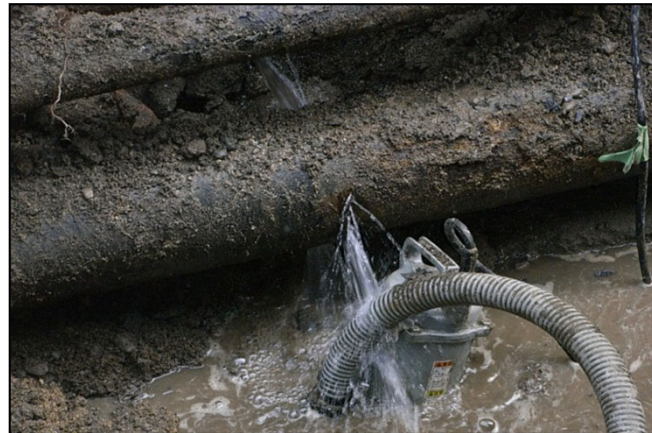
Rupture of aging water pipes
