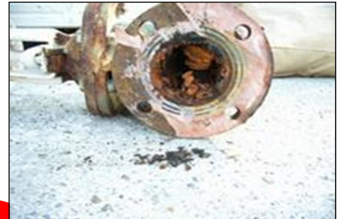
Red water due to aging, rusty water pipes
