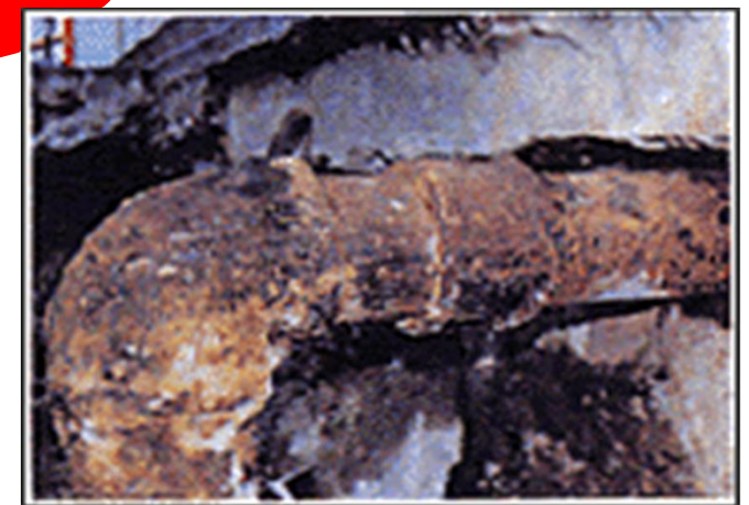
Aging gas pipes
