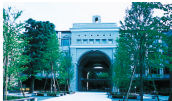
Yoshida South Campus Academic Center Bldg.
