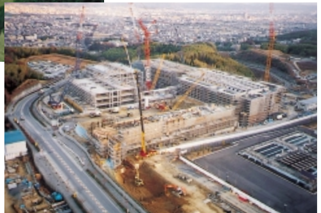
Cluster A under construction (December 2001)
