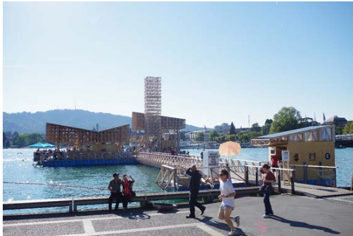
Floating Timber Pavilion, Zurich
