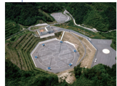
Area view of the middle and upper atmosphere radar (MU radar)
